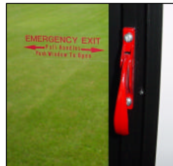
Figure 17: Egress Window Release Handle in Closed Position
