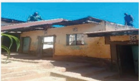
Orphanage roof leaks repaired
