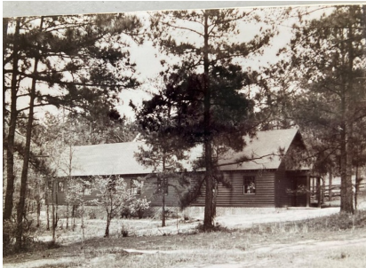
The parish's early church building, c. 1950s.
