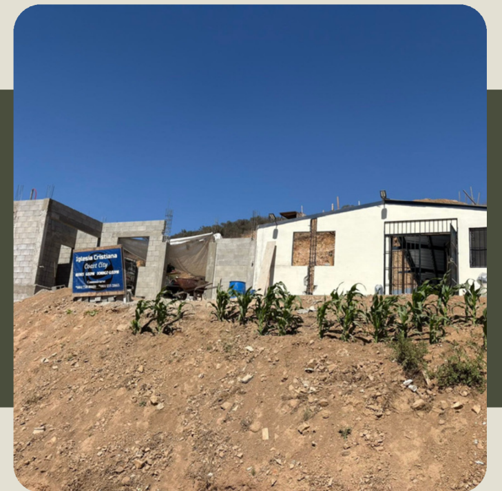
Coast City Tijuana Church Build in progress.
