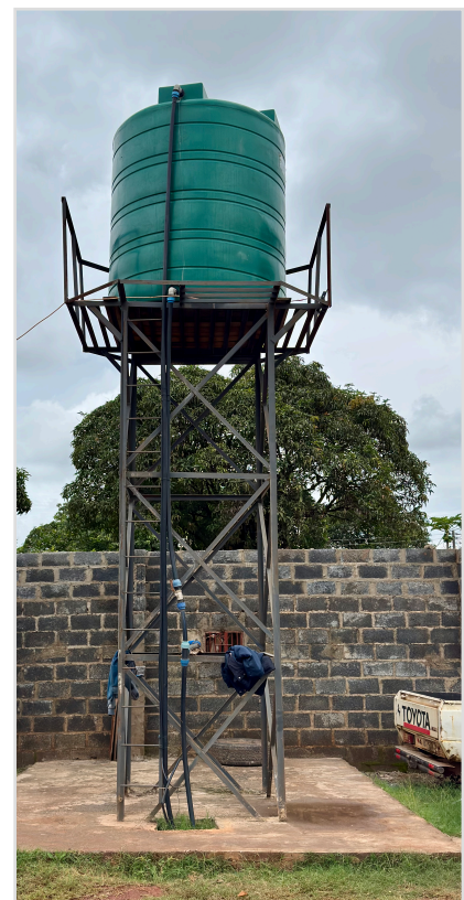
The borehole completed at Union Baptist
