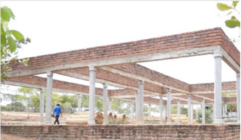
New and larger dining hall under construction.
